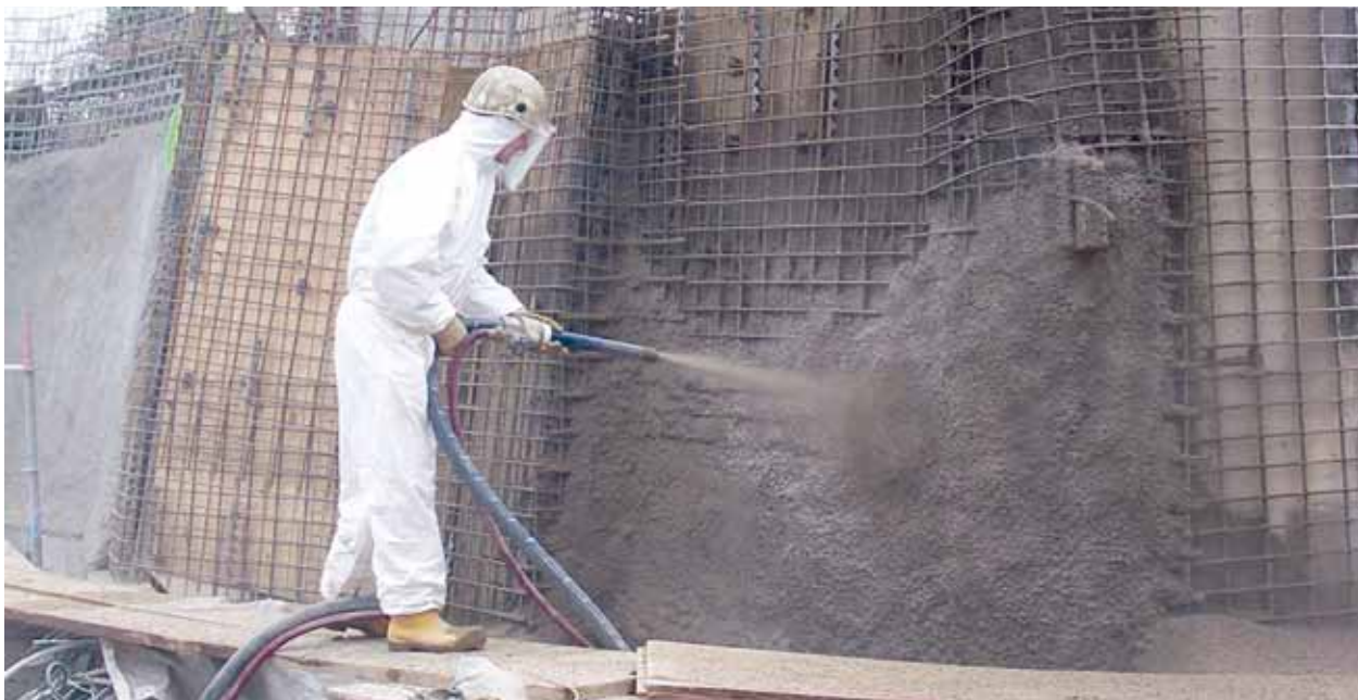
Sprayed Concrete Process
